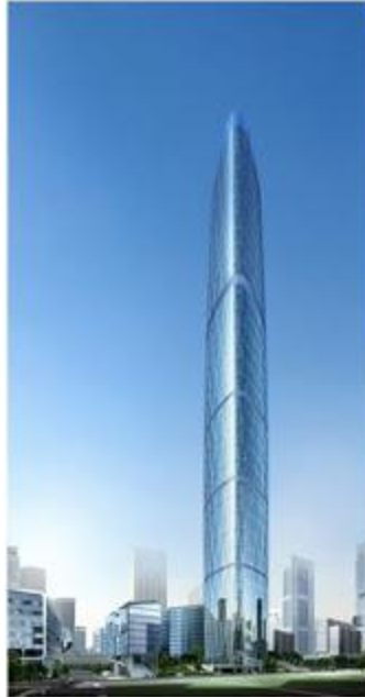
Figure 16: Guangzhou West Tower, China
