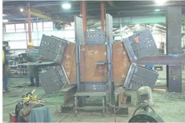
Figure 11: A Diagrid node after fabrication
