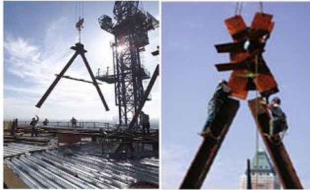
Figure 13: Diagrid Erection Process
