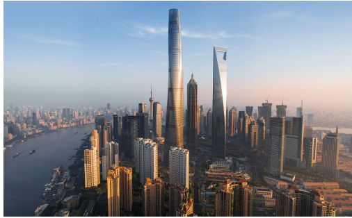
Shanghai Tower - Shanghai, China
