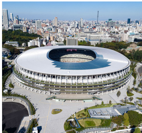
Japan National Stadium
