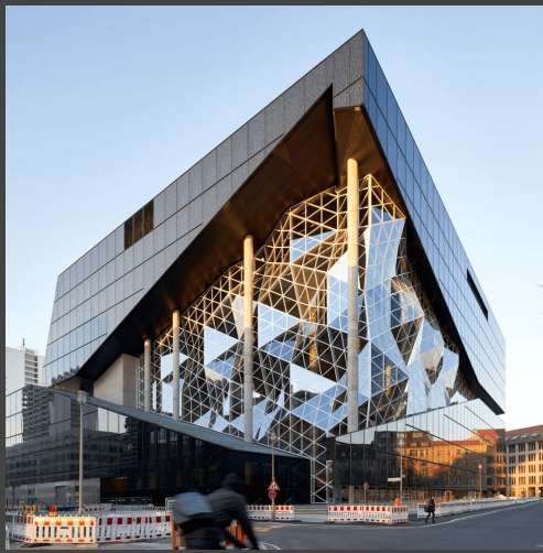
Axel Springer Campus Building
