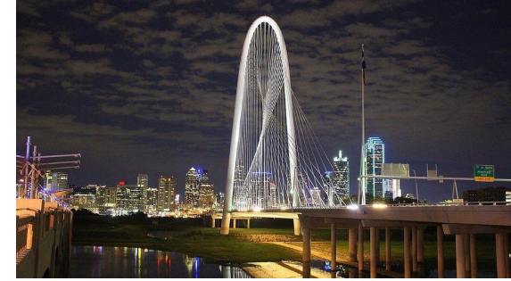
Margaret Hunt Hill Bridge - Dallas, TX
